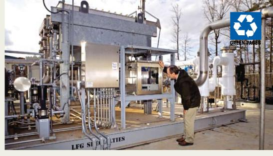
Interface Inc. pipes in methane gas from a nearby landfill in LaGrange, Georgia, to power one of its plant processes. Here VP of Engineering, David Gustashaw, monitors the gas analyzer. As methane is drawn off to fuel the factory, the entire landfill volume is drawn down, increasing its capacity and postponing the city's next landfill opening for an estimated fifteen years.
